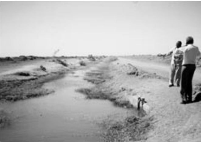
Gezira irrigation scheme. Siltation and weeds in small canals disrupt the flow. Photo: S. Mason 2001.
