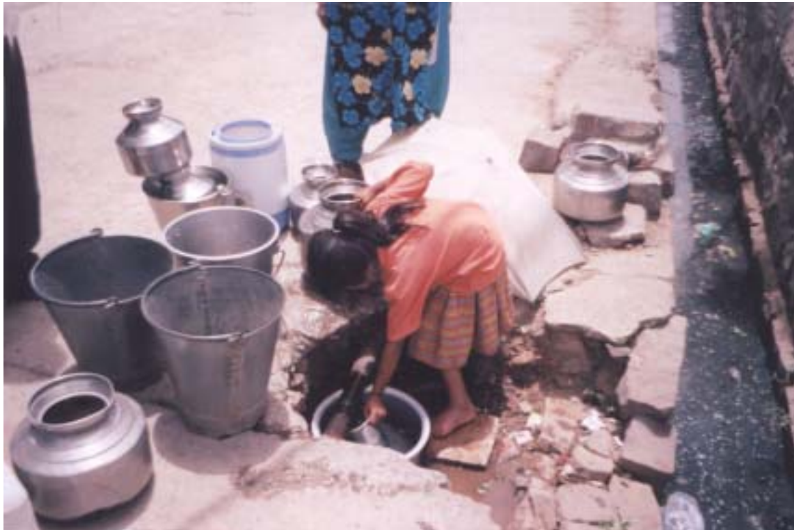
A Girl Child filling the buckets from leaking pipe in Bhopal
