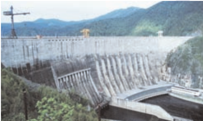
The International Commission on Large Dams (ICOLD) defines a large dam as being over 15 m high. The definition also includes dams between 5-15 m high with a reservoir exceeding 3 million cubic meters.
