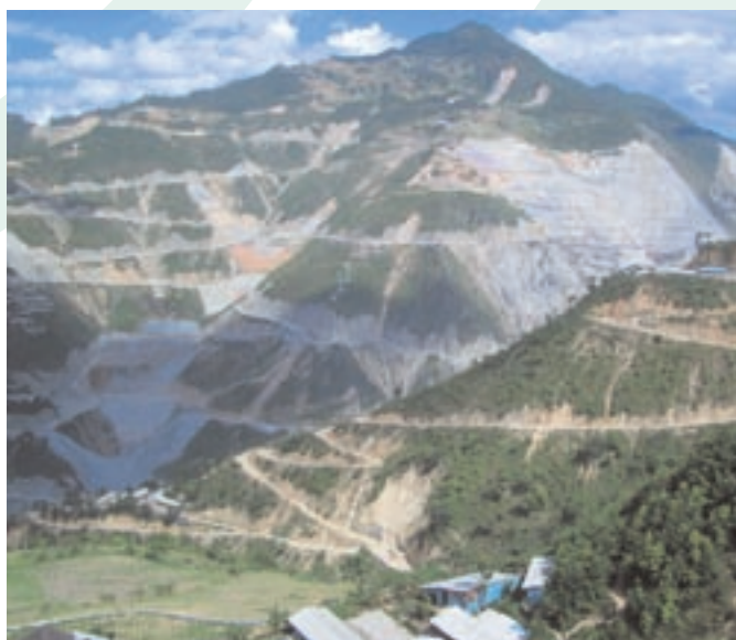
The building of access roads to the construction site of the Xiaowan dam on the Upper Mekong (Lancang) river in China has already caused considerable damage.
