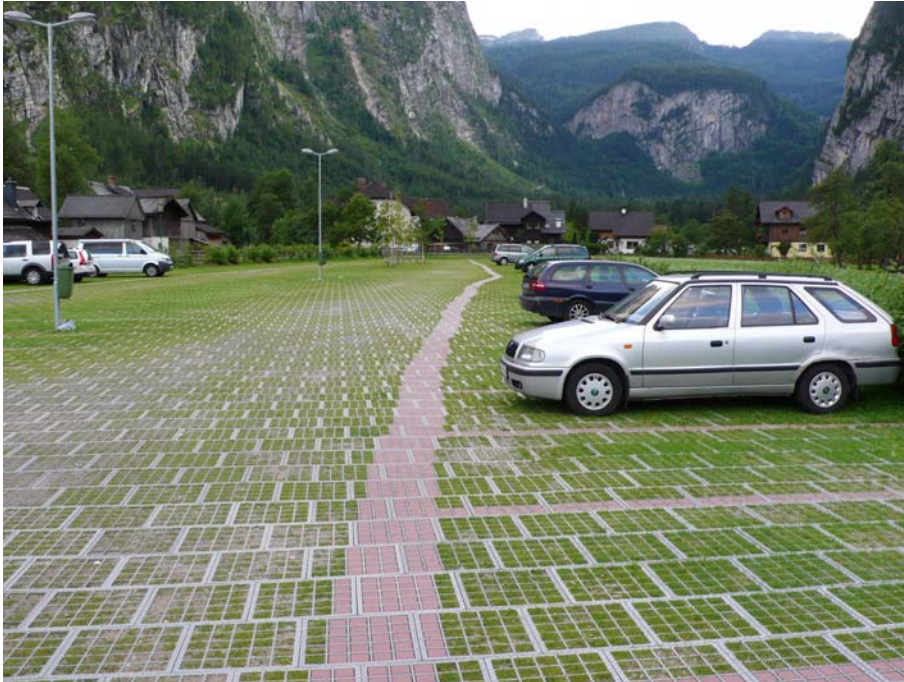
Figure 11. Another example for Sustainable Drainage Urban System (SDUS) for a parking lot avoiding runoff and facilitating infiltration to the aquifer. Hallstatt, Austria. Photo Ignacio Prieto.
