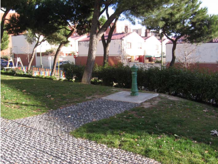
Figure 4. An example for Sustainable Drainage Urban System for a drinking public fountain spilling the effluents for a buried SDUS system so as to recharge the aquifer. Madrid.
