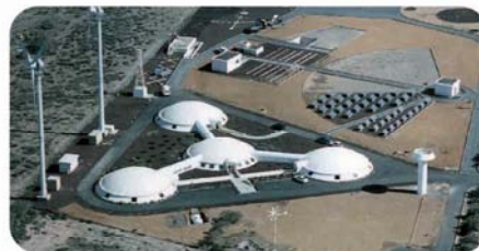
Reverse osmosis waste water treatment plant.
