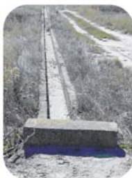
Drainage ditch on a hillside. The collection of rainwater reduces erosion and enables greater use of the runoff water. Navarre. (Photo: TRAGSATEC).
