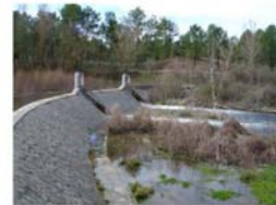
Dam for MAR on the river Pirón, Shire of Carracillo, Segovia (Spain).
