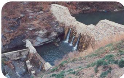
Dyke in a torrent in Sierra Nevada (Granada). It laminates the peak flow volume and increases infiltration (Photo: TRAGSATEC)
