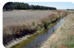
Picture of the infiltration pond and artificial recharge channel of the Cubeta de Santiluste facility (Segovia).
