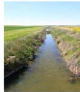
Recharge channel in Santiuste, Segovia (Spain).
