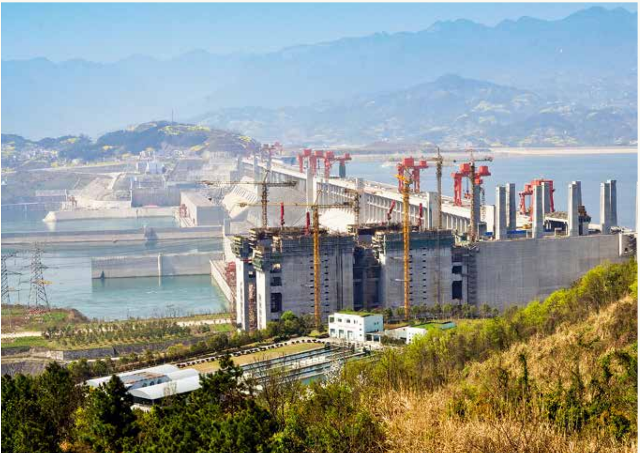
The Three Gorges Dam, spanning the Yangtze River in Hubei province, China, is the world's largest power station.
