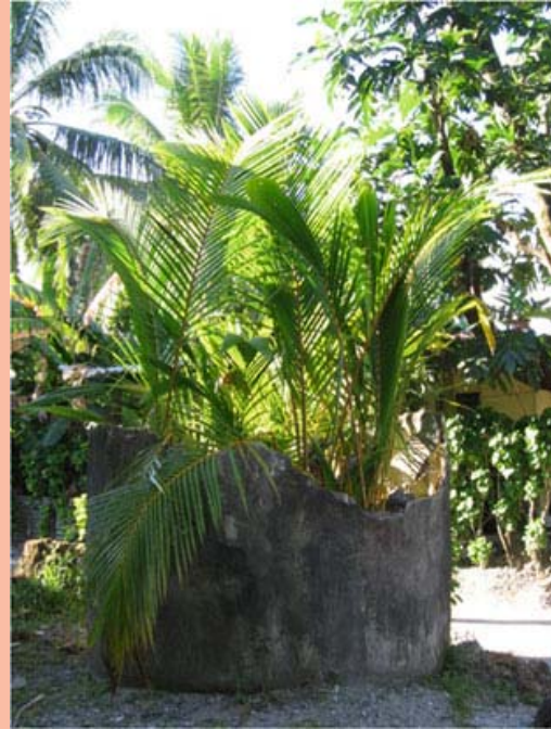
Box Fig. 1.5a.4 Broken tank: Rainwater catchment tanks are prone to cracking and breaking when not maintained and kept full of water. A broken tank on Funafuti Atoll collects organic material and makes a fertile home for new palm growth (Photo credit: Heather Lazrus)
