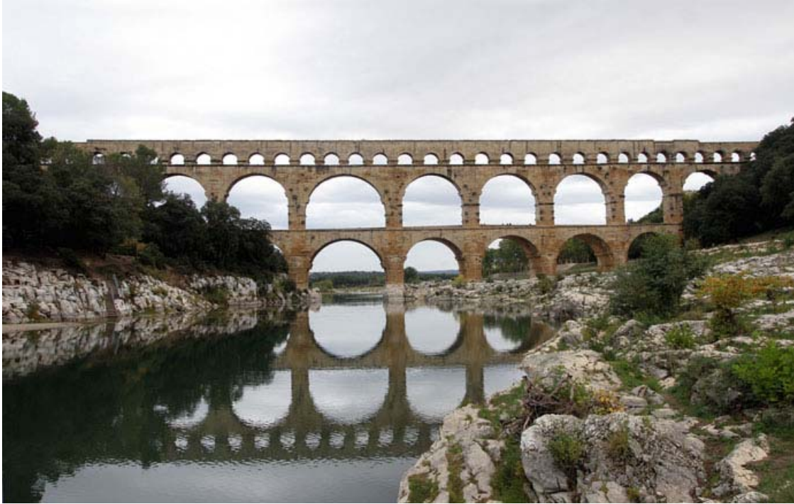
Fig. 1.1.2 The Pont du Gard is part of a 50 km aqueduct in southern France constructed by the Romans in the first century A.D. It was added to UNESCO's list of World Heritage Sites in 1985 (Photo credit: Armin Kübelbeck, http://commons.wikimedia.org/wiki/File:Pont_du_Gard_01.jpg )
