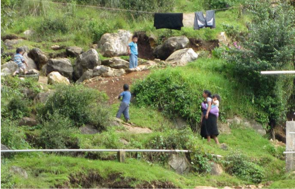
Fig. 2.5.4 Pipes carrying water from El Pinar to La Hormiga (Photo credit: Ameyali Ramos Castillo)
