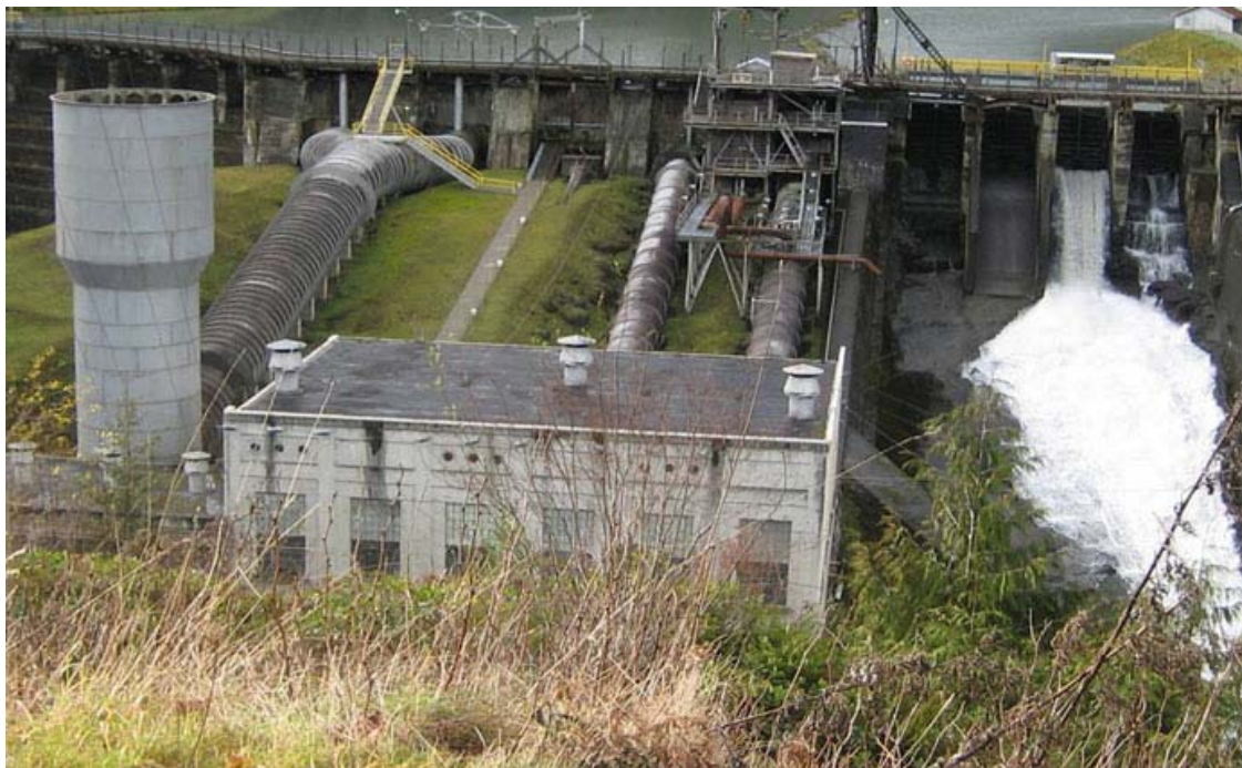
Fig. 4.6.1 The Elwha dam, 2007 (Photo credit: Colleen Boyd)
