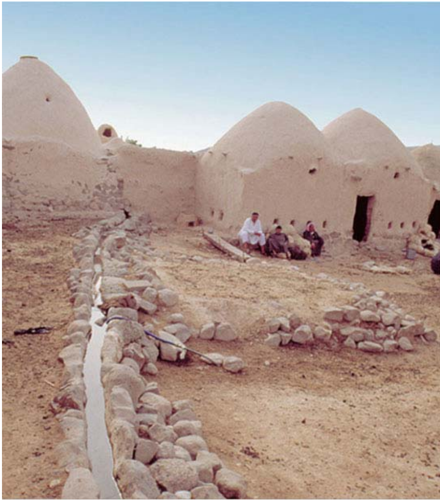
Fig. 2.3.2 Open channel in qanat community in North West Syria (Photo credit: Joshka Wessels)
