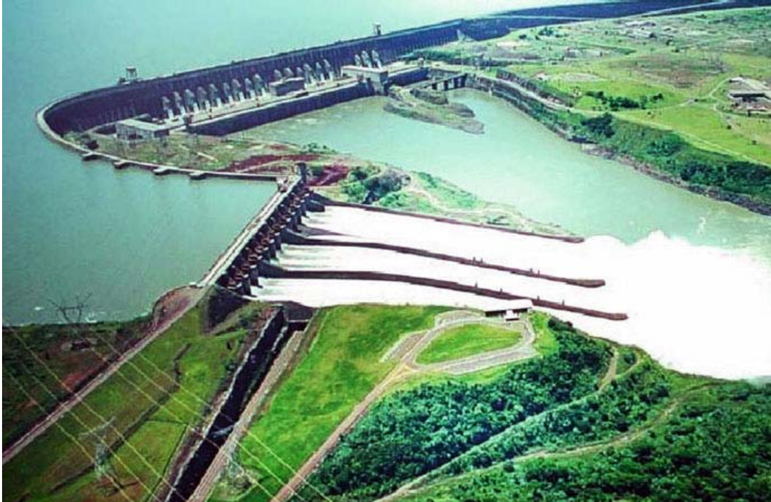
Fig. 1.1.7 Itaipu dam during release (Photo credit: Angelo Leithold 2005)
