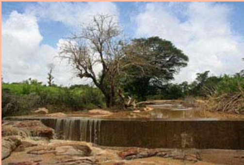
Box Fig. 2.2a.3 A sand dam during the wet season (Source: NWP 2007)
