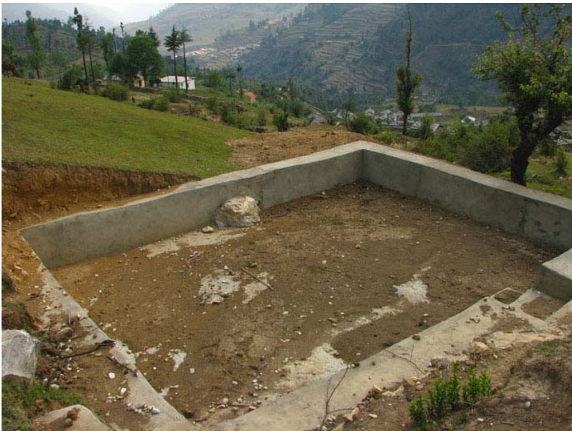
Fig. 5.1.2 A chaal in Thaandi village, Dunda block, Uttarkashi, constructed with NREGA funds (Photo credit: A. Acharya)
