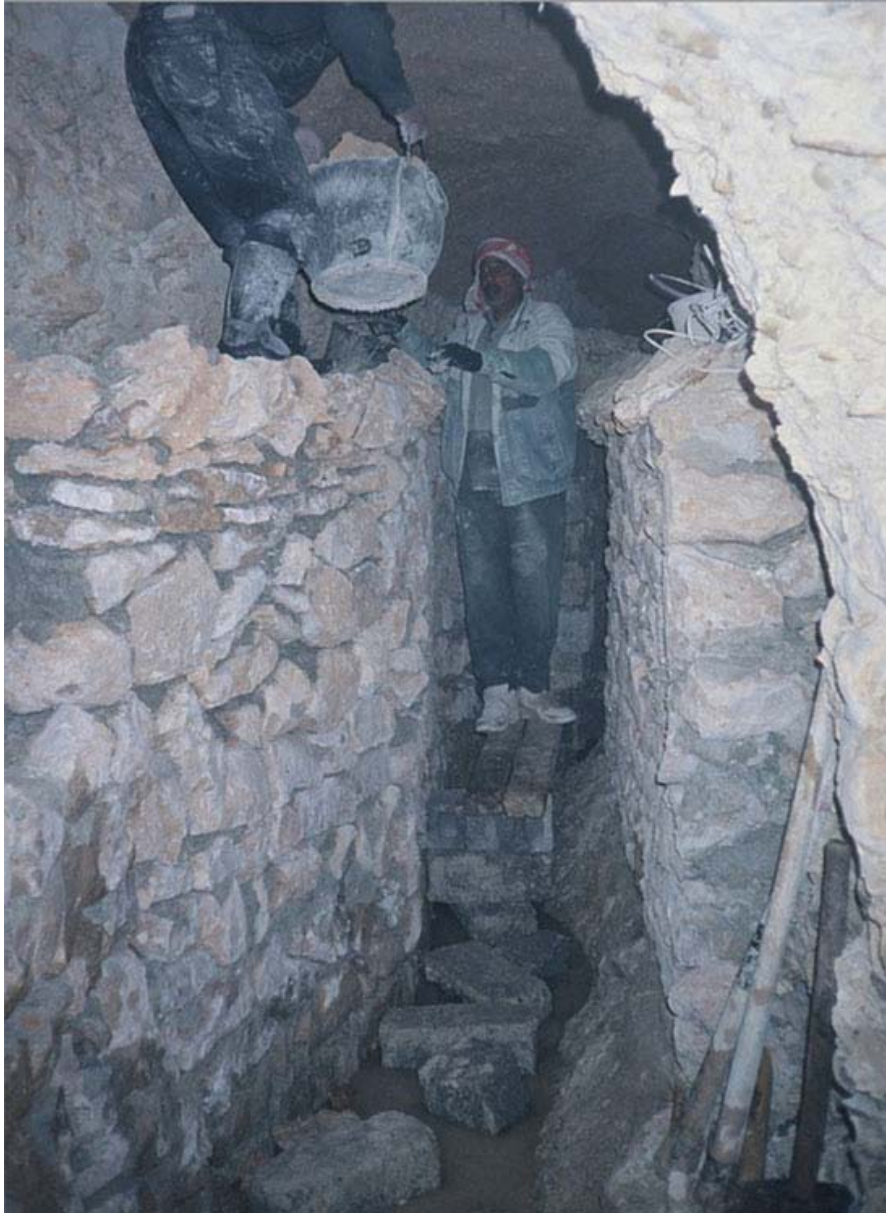
Fig. 2.3.3 Users renovating and cleaning their qanat in South West Syria (Photo credit: Joshka Wessels)
