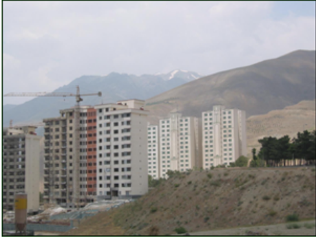
Figure 5: more buildings at city limits
