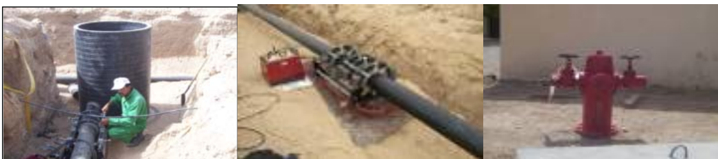
Photos of Phase 2: Water distribution
