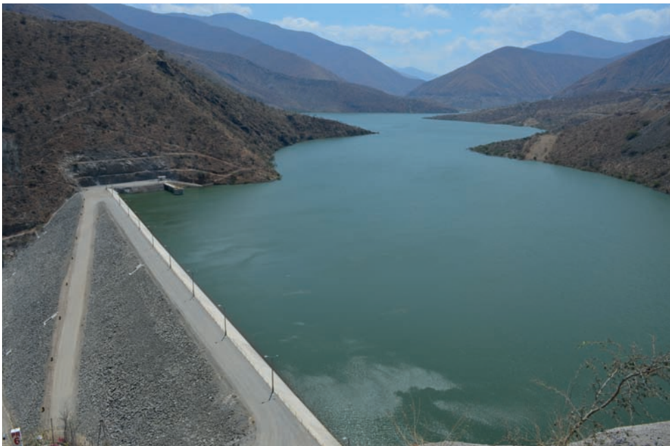
Figure 4 Limon Dam and reservoir. It was built on the Huancabamba River, in the Amazon Basin, to store water and divert it to the Olmos River, in the Pacific Basin (Kuroiwa, August 12, 2012).
