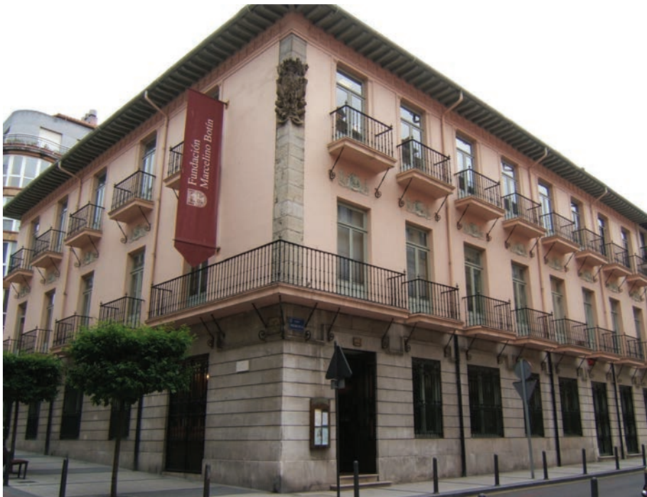
Headquarters of the Marcelino Botin Foundation in Santander (Spain)
