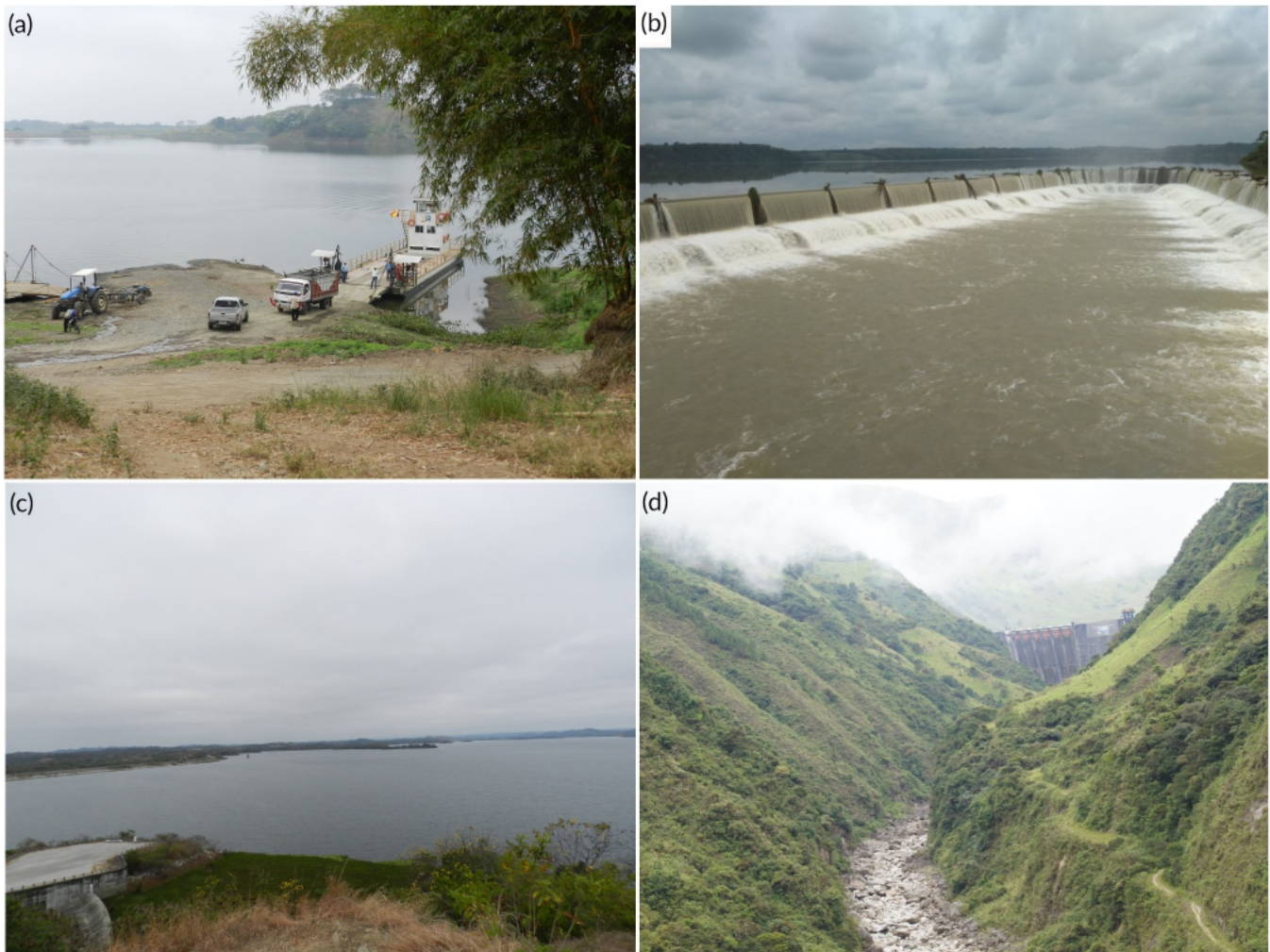
FIGURE 7 Dams have been constructed in rivers throughout Ecuador and more dams are planned. (a) View of impoundment formed by Daule-Peripa Dam, upper Guayas basin (western Ecuador). (b) Dam in the Baba River, Guayas drainage basin (western Ecuador). (c) Impoundment formed by the Chongon Dam outside of the city of Guayaquil (western Ecuador). (d) Daniel Palacios Dam (Paute Integral Hydroelectric Complex) showing river without water (Andes)
