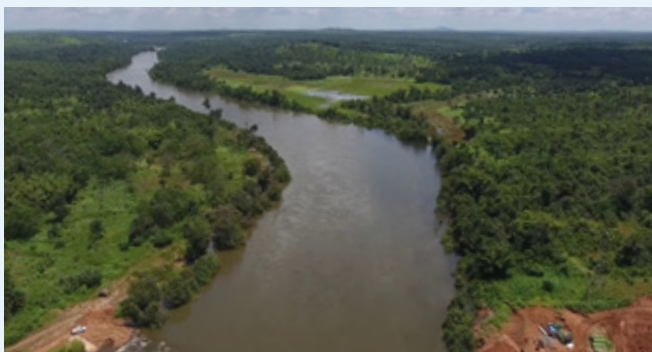
Rokel River at Rogbere bridge, Sierra Leone. Photo credit: NWRMA.
