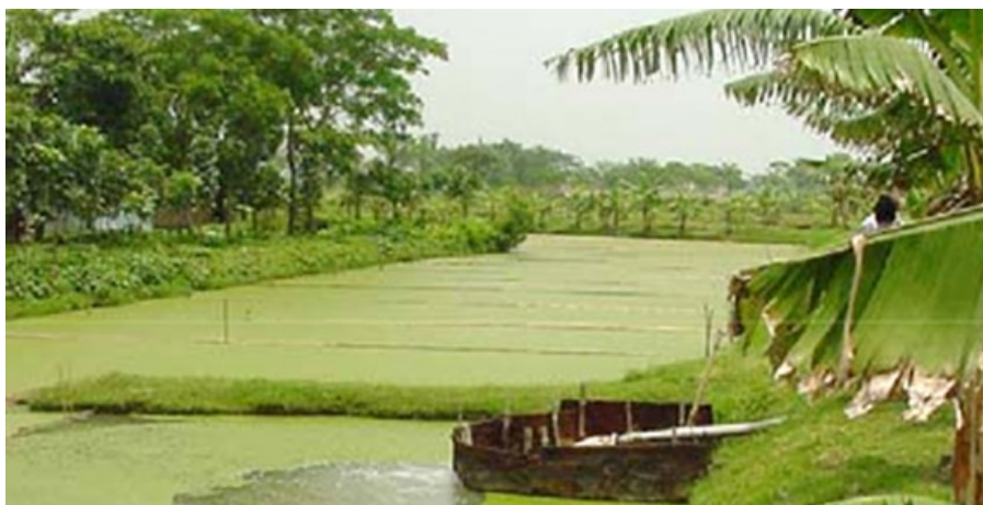
Figure 2: Duckweed-covered plug-flow treatment system in Mirzapur, Bangladesh.
